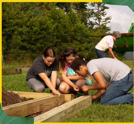
Photo courtesy of Rabun County School District
